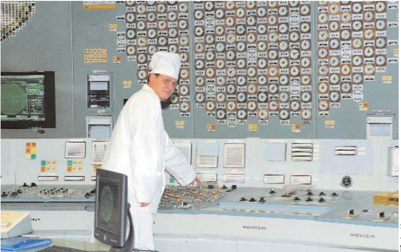
This is it – the important shutdown button is being pressed by senior reactor control engineer Alexander Beschastnov.
